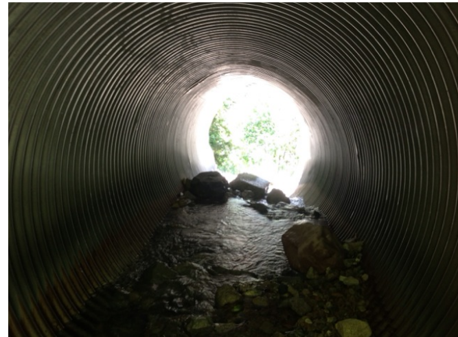
looking through culvert
