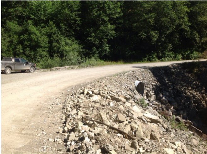
Approach from Right Bank when facing downstream
